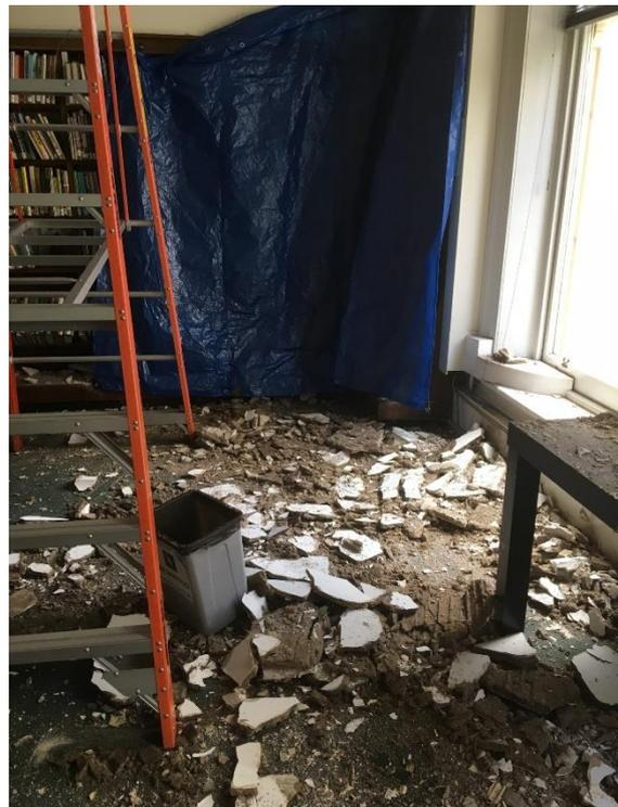
WorkSafe has cleared the area for access for repairs, large fans are drying the ceiling out, and scaffolding should be erected this week. We are working with insurers and plasterers, and it is likely that most of the ceiling section over the affected area will have to be removed and replaced.
